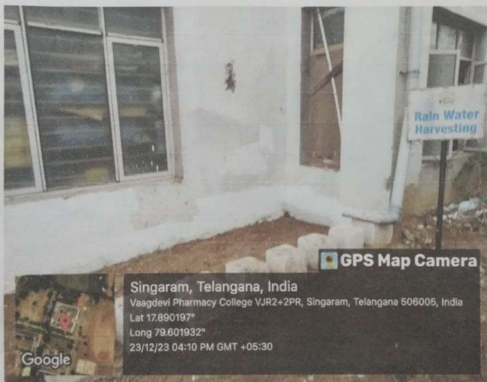
Rain water harvesting structure
